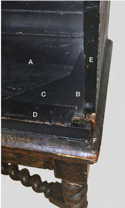
**Figure 9** The assembly of the stand and the upper case. The right door has been removed to show the bottom and the cleat of the cabinet's interior. A= bottom, B= cleat, C= corner block, D= front rail, E= side panel, F=profile along the top of the stand.
